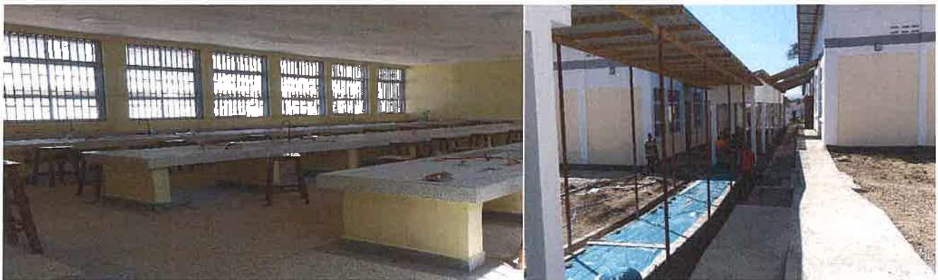
Figure 5: Construction of workshops/laboratories
