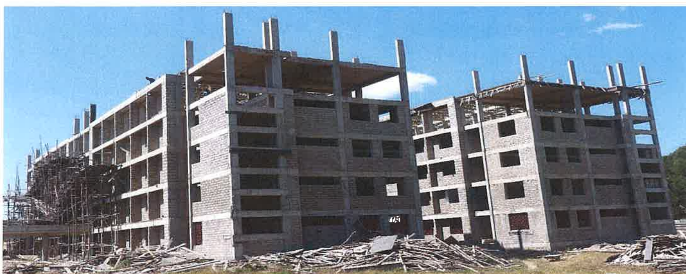
Figure 6: Construction of students' hostel
